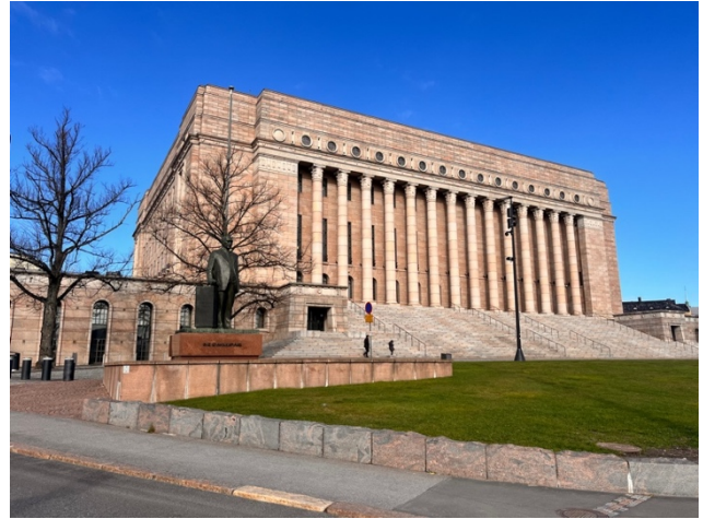
Parliament building in Helsinki
